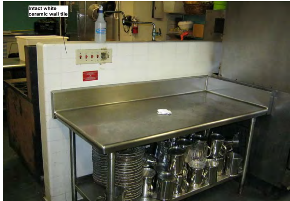
Photograph 13: View of intact lead-containing white ceramic wall tile in the 2 nd floor kitchen of the restaurant building.
