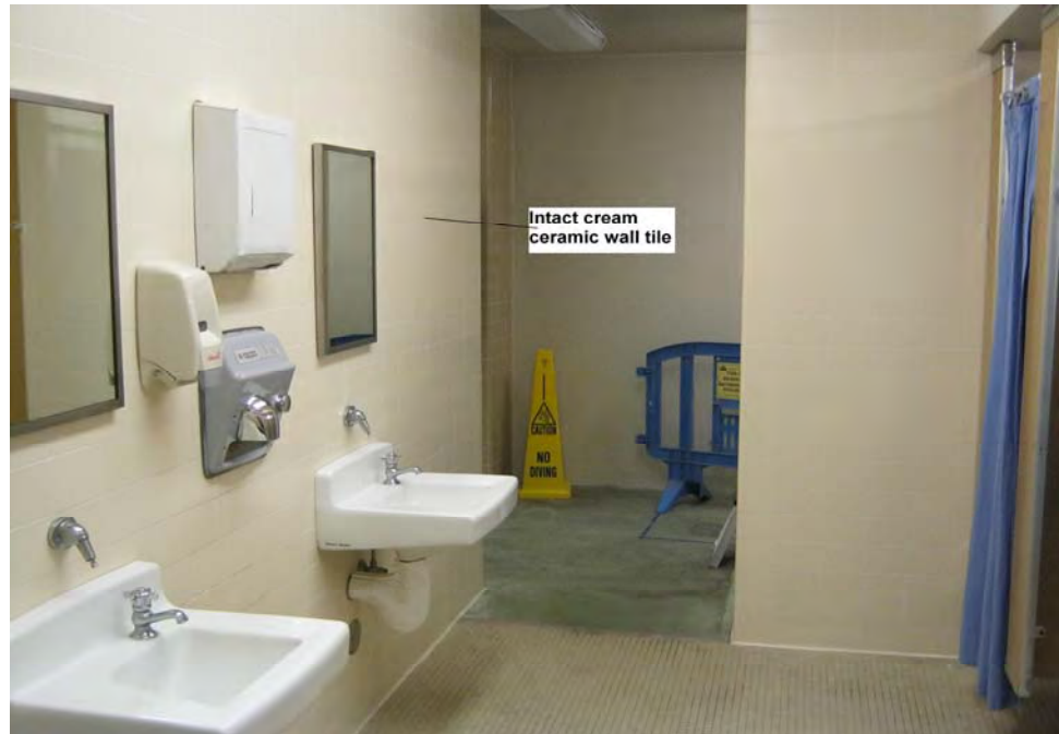
Photograph 29: View of intact lead-containing cream ceramic wall tile in the women's executive locker room in the locker rooms and office building.
