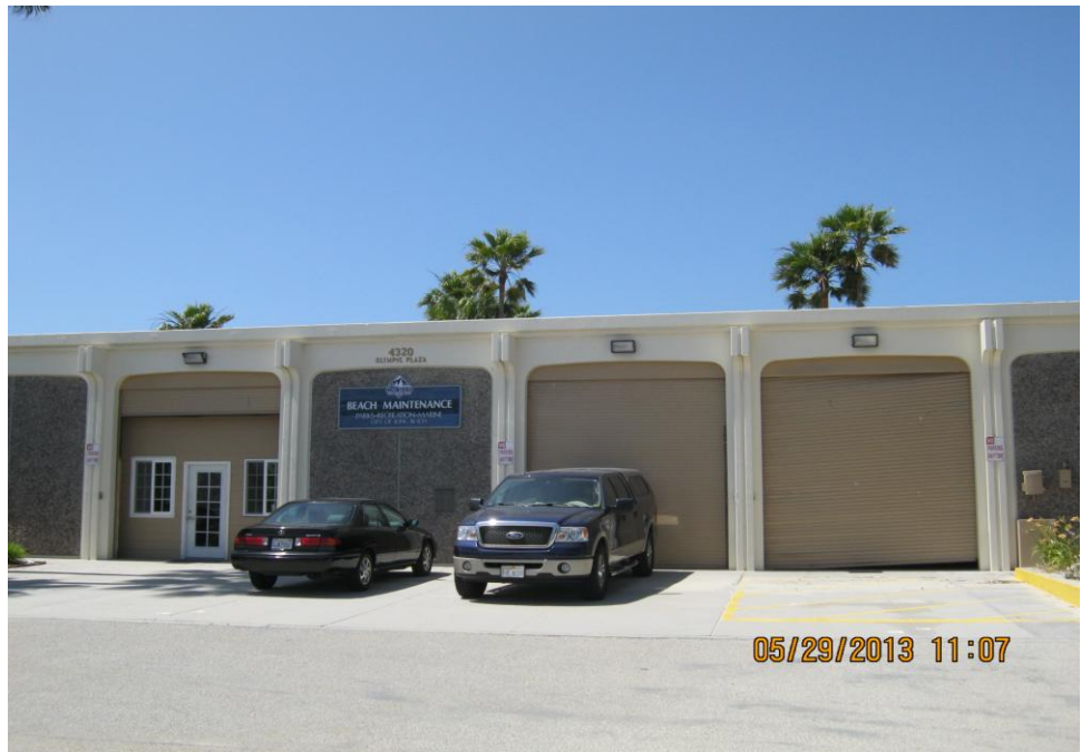
Photograph 15: Looking at the City Beach Maintenance building located east of the site.
