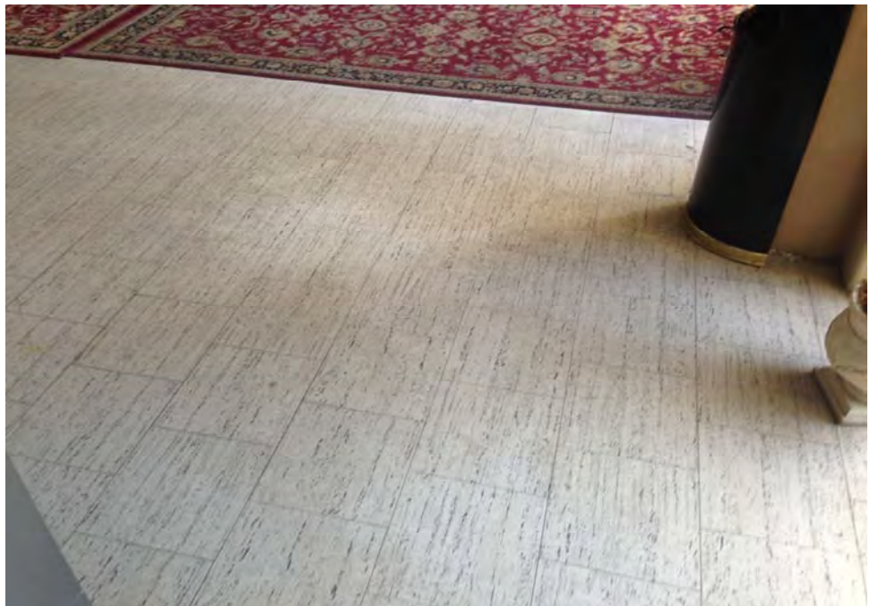
Photograph 8: View of asbestos containing vinyl floor tile and mastic on the second floor of the restaurant building.
