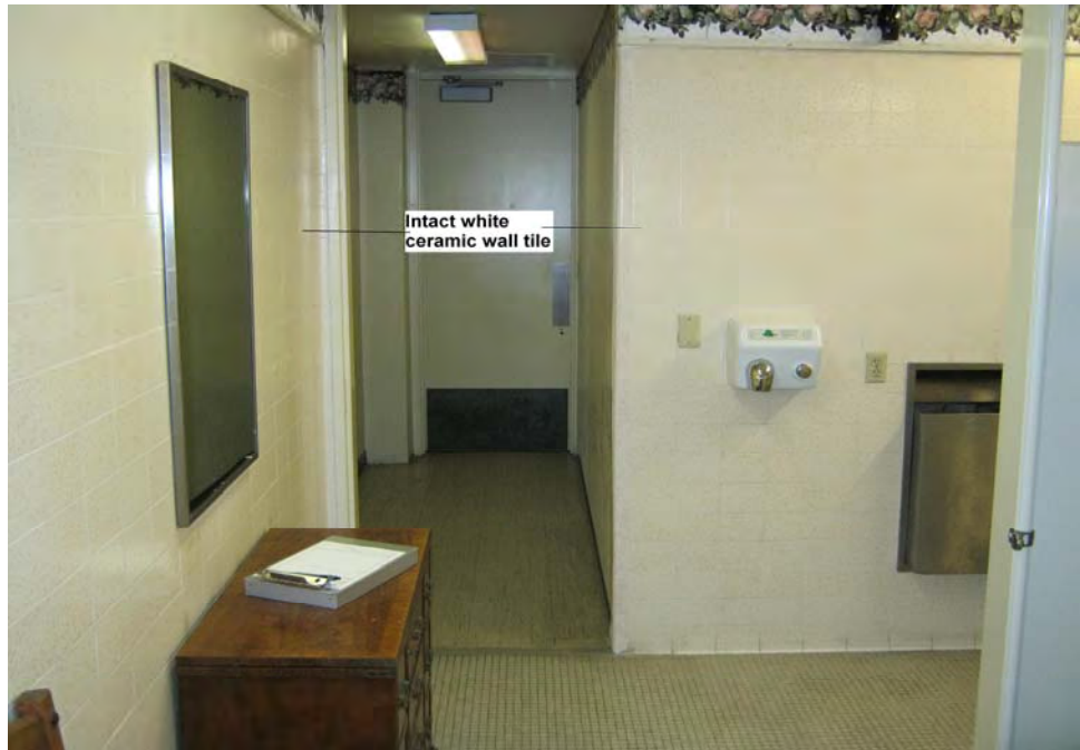
Photograph 15: View of intact lead-containing white ceramic wall tile in the 2 nd floor women's restroom of the restaurant building.
