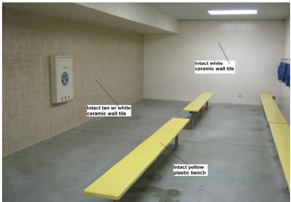
Photograph 28: View of representative intact lead-containing white and tan with white ceramic wall tile, and yellow paint on plastic benches in the women's, men's women's executive, men's executive, and women's employee locker rooms in the locker rooms and office building.
